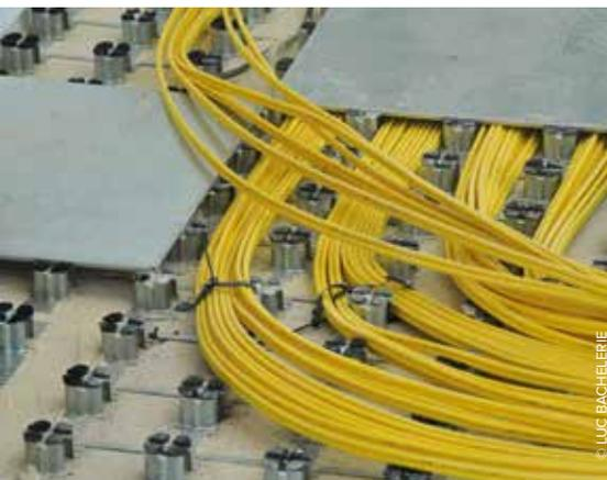
▲ LE SYSTÈME DE PLOTS INTERCELL D'INTERFACE EST COLLÉ SUR LE SUPPORT. LA CONFIGURATION DES PLOTS DÉTERMINE UN RÉSEAU POUR LA GESTION DES CÂBLAGES.
